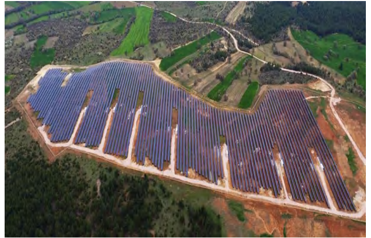
Location : Gediz ,Turkey Capacity : 8MW
