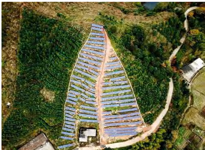
Location : Gansu, China Capacity : 500KW
