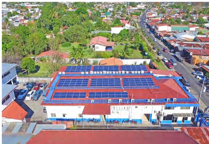
Location : Costa Rican Solar Project Capacity : 45KW
