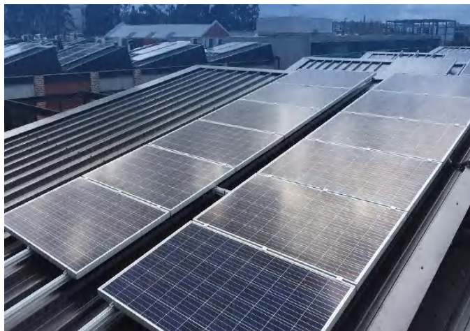
Location : Kuala Lumpur, China Capacity : 20KW
