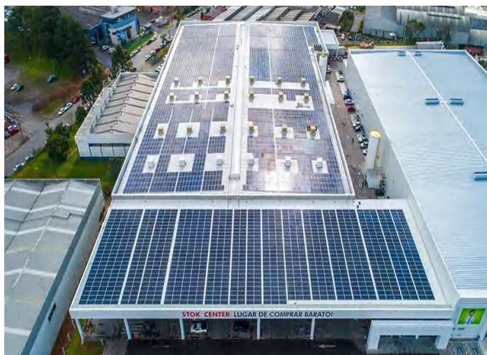
Location : Caxias do sul, RS-Brazil Capacity : 1.4MW
