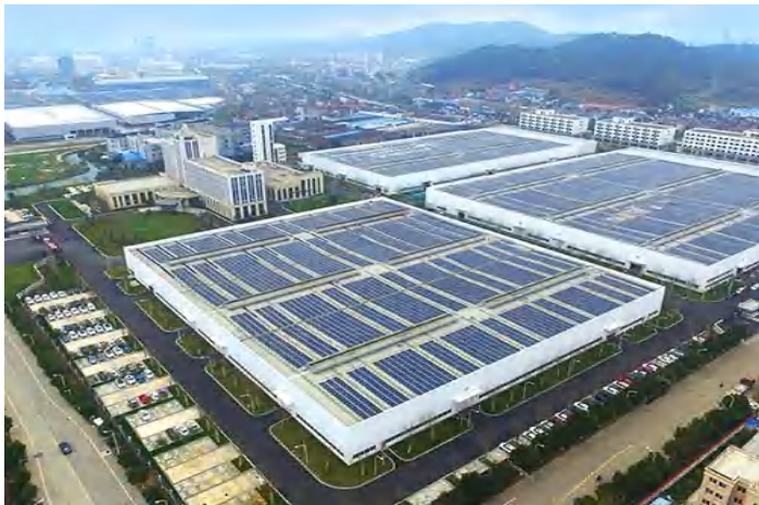
Location : Munich, Germany Capacity : 5.5MW
